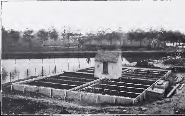
Installation for the University Hospital, Groningen, Holland.
